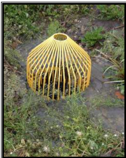
Yellow “Bar Guard” covers tile inlet. This protects the tile from debris entering into the tile and potentially plugging up the underground tile system
